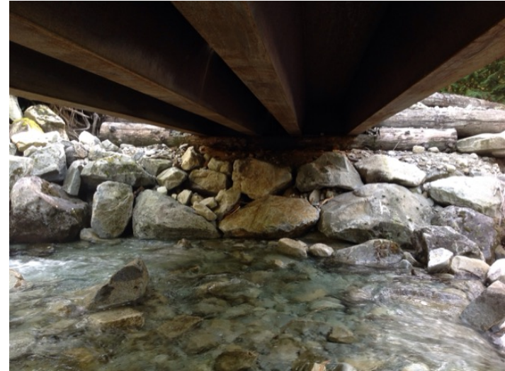
Left Bank Abutment when facing downstream
