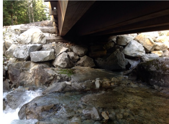
Right Bank Abutment when facing downstream
